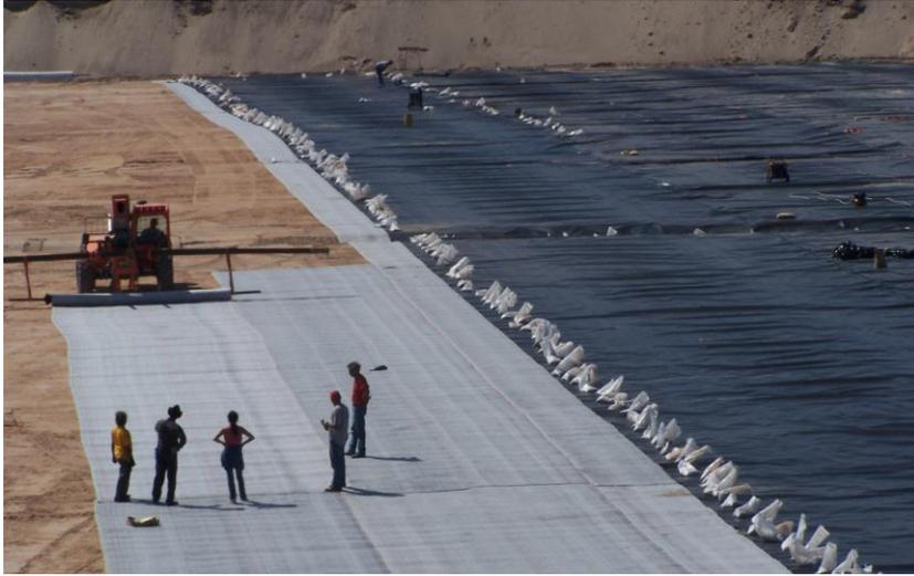
Why is it okay to throw the pills in the trash? Since the early 1990's U.S. landfills have been designed and built by environmental engineers with several liners in place to prevent groundwater contamination. In our area, we use two feet of compacted clay, a geothermal textile liner, a 60 mil high density polyethylene liner and two feet of sand on top to protect the engineered liners from the heavy equipment that crushes
